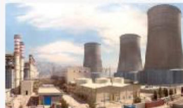
Zahedan Combined Cycle Power Plant
