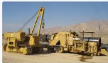
Mahshahr - Torbat Heidarieh Gas Transfer Pipes
