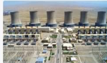
Damavand Power Plant
