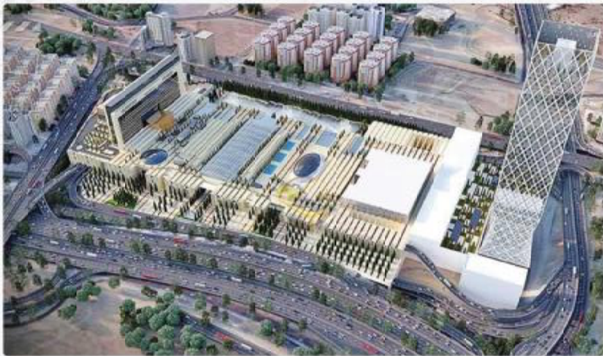
Iran Mall Electrical Substations MV & LV Panels
