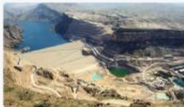
Gotvand Dam and Hydroelectricity Power Plant
