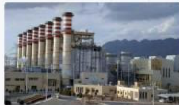
Kerman Combined Cycle Power Plant
